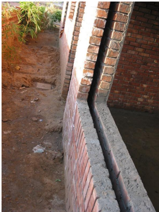
Fig.7. Cavity Wall
