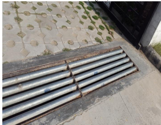
Fig.11. A steel pipe arrangement made at sector-17, Panchkula.
