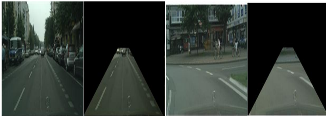
(a) Smooth and good road surface.
