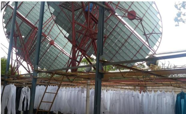
Fig.2. Solar Thermal system using scheffler collector at Gajraj Drycleaners
